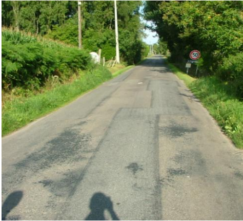
A typical French village road with surfacing maintenance applied when and where needed.
