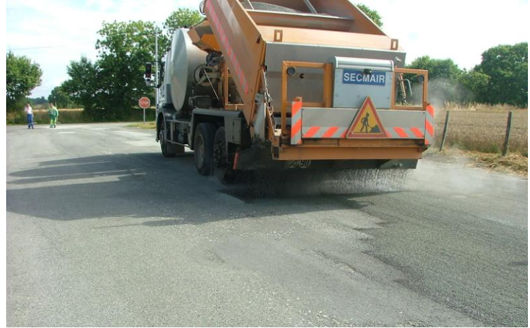
Local Chip Seal contractors take care of all Chip Seal surfacing needs in their area. In most cases they have a small outfit of one or two machines.
