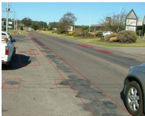
Example of a road surface in Australia that would benefit from surface dressing patches.
